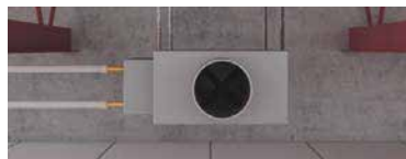
HYDRONIC VAV BOX APPLICATION
